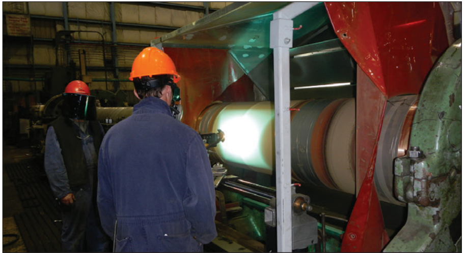
Advances in thermal coating processes means repairs to components like tail shafts can be done quicker than re-manufacturing and will extend the life of the repair.
