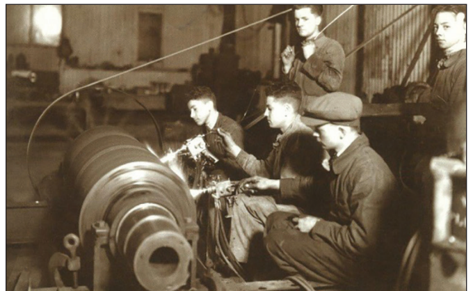
The old days — problems with temperatures, alloy quality and bonding made early thermal coatings an unattractive solution to most repairs.
